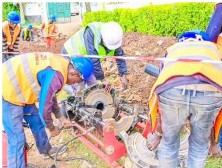
Plumbers joining 45 kilometers of pipes to supply water to Bureti Sub County.
