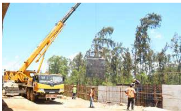
A section of the Mombasa-Mtwapa road currently under construction.
