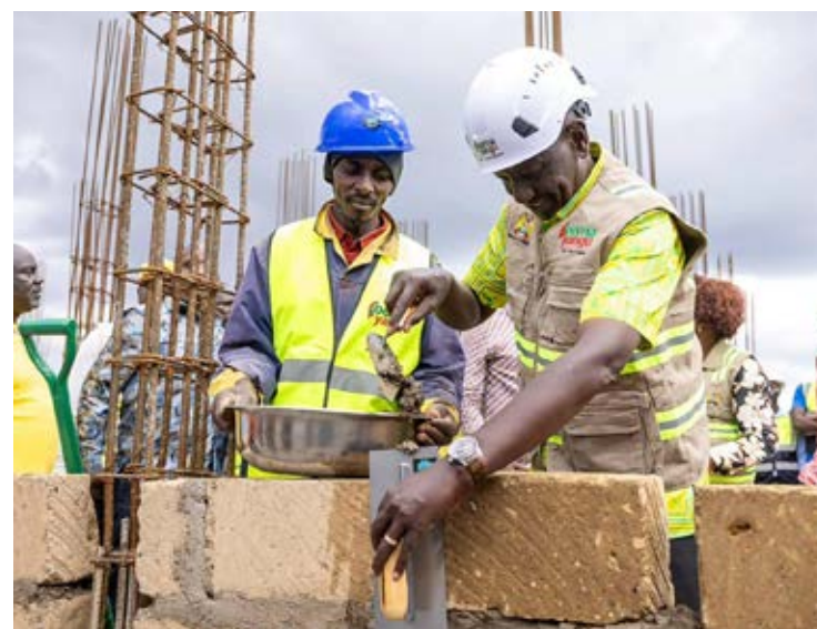
President William Ruto, right, in white helmet laying a foundation stone for a 50-bed capacity inpatient block at Meteitei Sub-county hospital in Tinderet Sub-county in Nandi.
