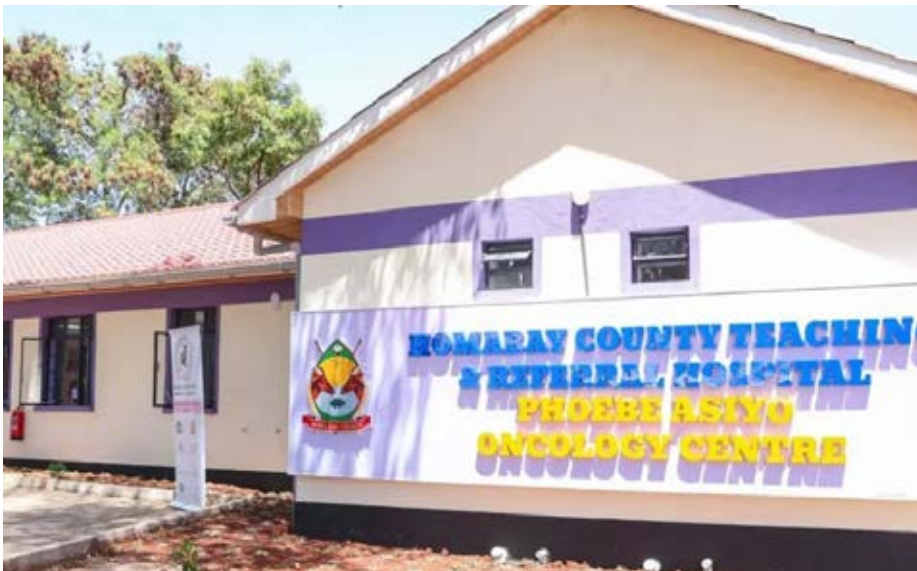
The newly launched Mama Phoebe Asiyo Centre in Homa Bay County. The centre will bring cancer diagnosis and treatment closer to the residents. Photo/ Sitnar Omar.
