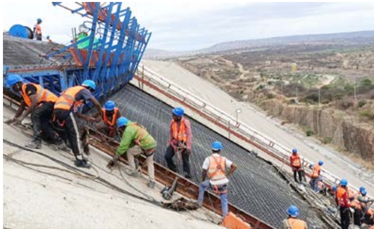
Workers at the Thwake Multi-purpose Dam who resumed working on the concrete Phase.
