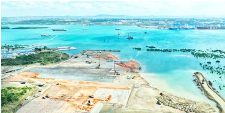
Ongoing construction of a new berth at the Mombasa Special Economic Zone (SEZ) in Dongo Kundu
