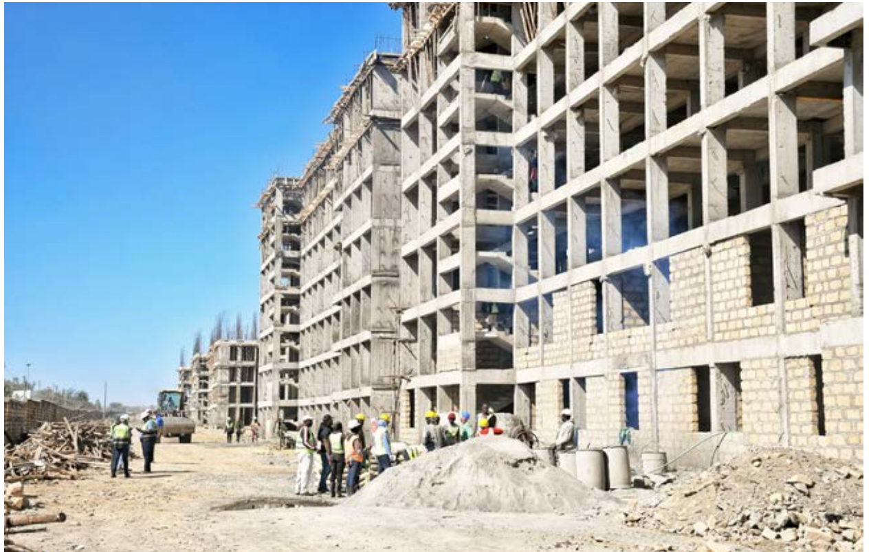
Affordable housing project at Karagita Estate in Naivasha under construction. The project has created job opportunities for local youth and micro, small and medium enterprises, stimulating the local economy. Photo by Erastus Gichohi.
