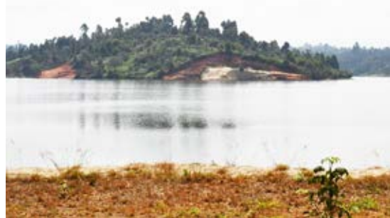
A section of the Karimenu dam. Photos by Annrita Mutembei.
