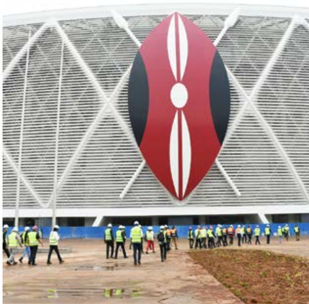
ongoing works at Raila Odinga International Stadium in Nairobi
