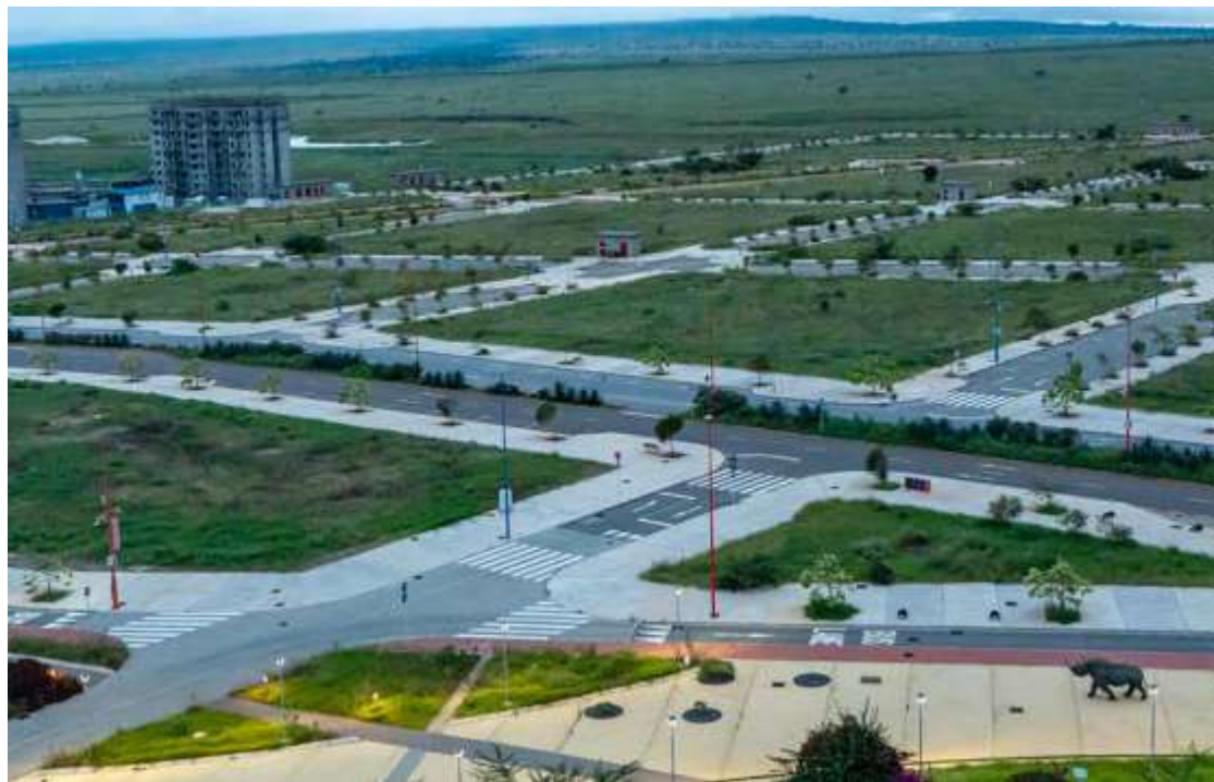
Road infrastructure at Konza City
