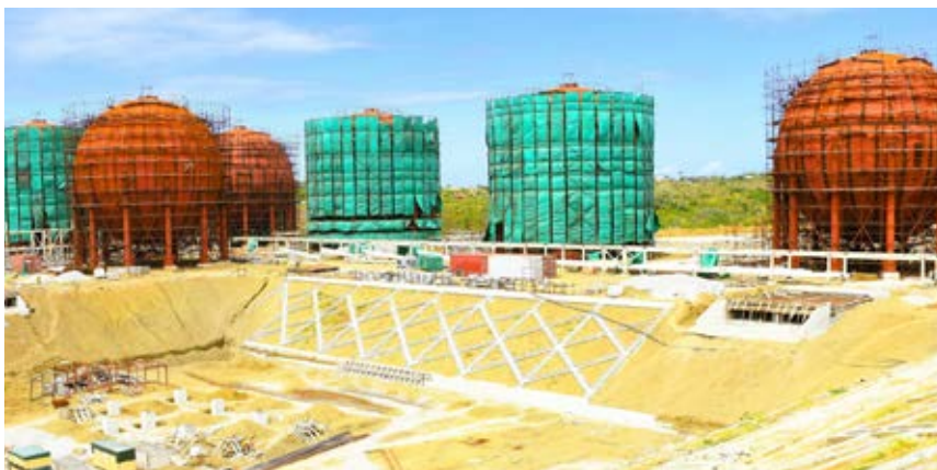
A general view of the Taifa Gas LPG Terminal at the Dongo Kundu Special Economic Zone in Mombasa. The massive energy project is nearing completion.
