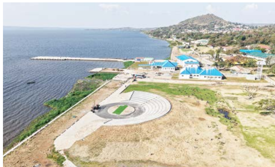
Aerial view of Homa Bay Pier Project. The new facility is expected to transform Homa Bay into a strategic transport hub to unlock regional trade.
