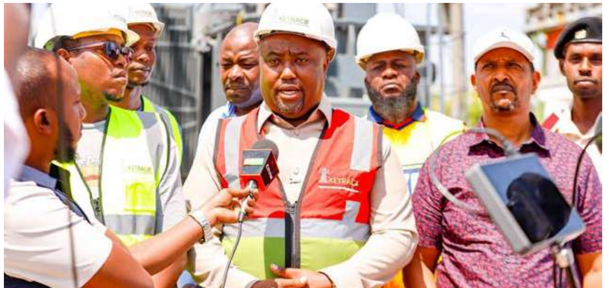
Energy PS Alex Wachira speaks at the Garissa Kenya Power substation after inspecting the progress of the commissioning of a new 23 MVA transformer.
