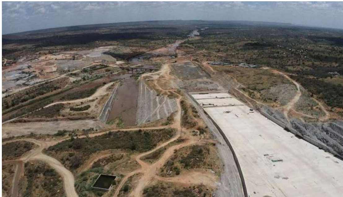
Thwake Dam, pictured, is expected to secure food production, protect millions of people from drought alongside powering new industries in Lower Eastern Kenya.
