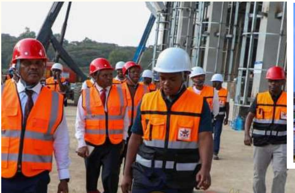
Major-General Peter Limo conducts an inspection of the ongoing construction of the Raila Amolo Odinga International Stadium, formerly Talanta Stadium, at the Talanta Sports Complex last Friday. The 60,000-capacity stadium (right) is nearing completion.
