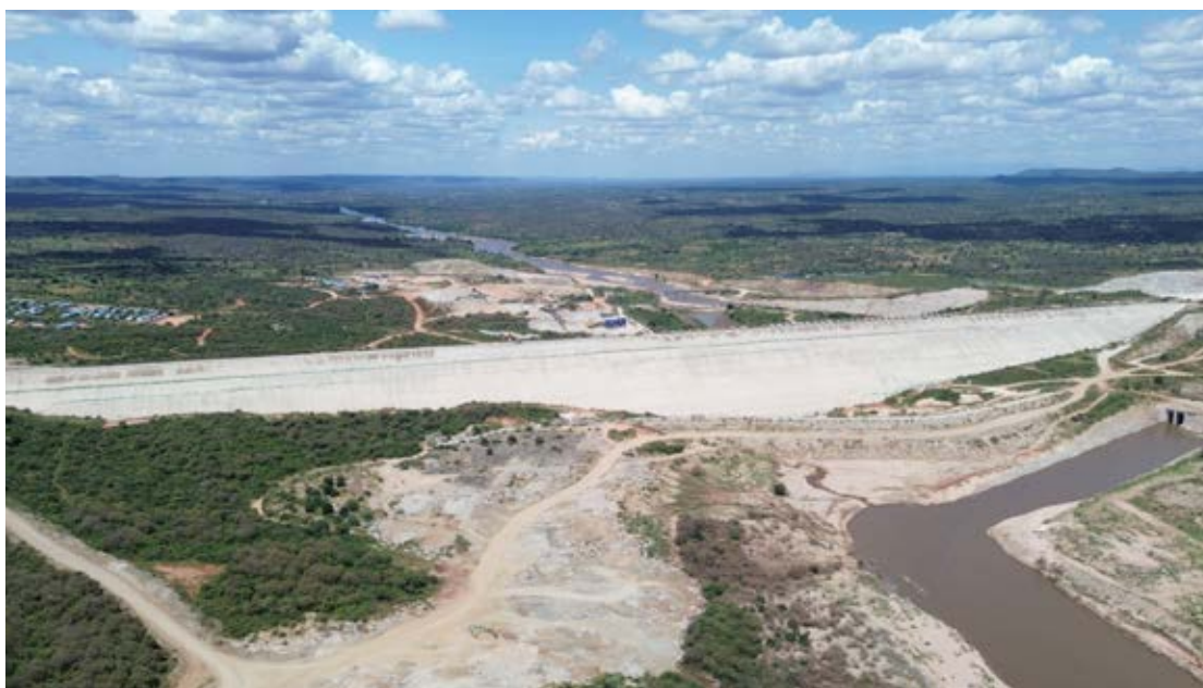
An aerial view of Thwake Dam that is expected to benefit 1.3 million people in Makueni, Kitui, and parts of Machakos counties when complete next year.
