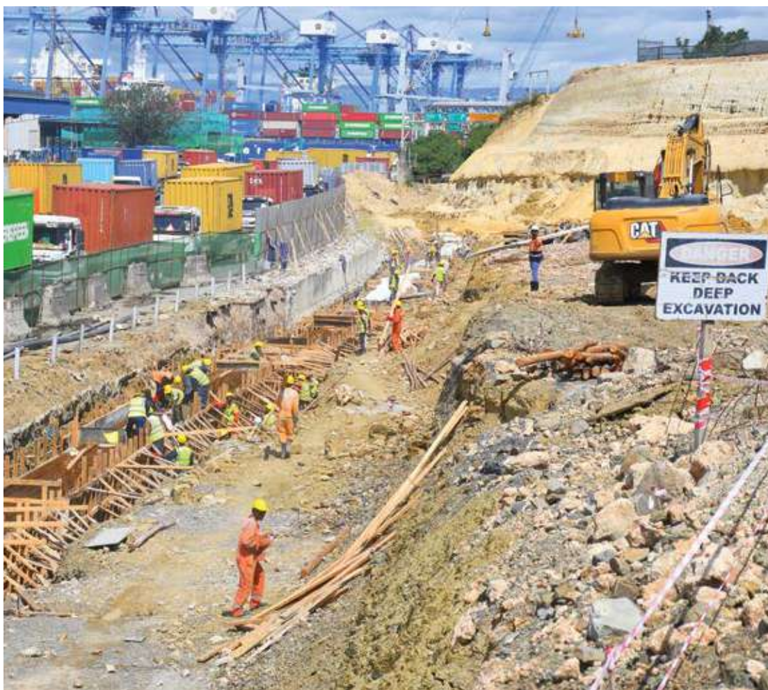
A section of the ongoing construction of the proposed widening of the port road from the gantry workshop to gates 18 and 20 at Kenya Ports Authority (KPA), Mombasa. PHOTO: ANDREW HINGA
