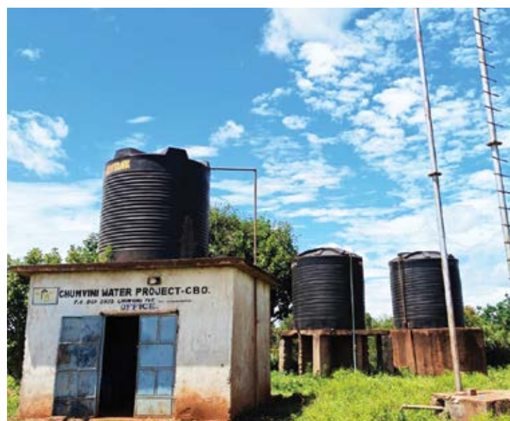
Water storage tanks at Chumvini Water Project in Taveta Sub-County, that have remained dry for over two years, is set to improve following the launch of the Sh400m Kenya Off-Grid Solar Access Project (KOSAP).
