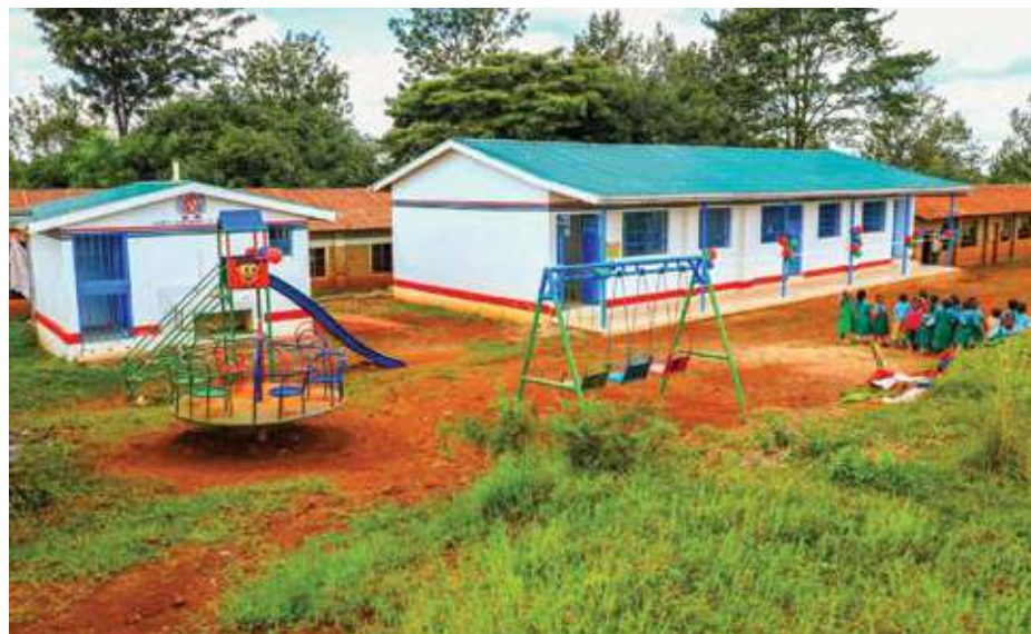
Learners interacting outside the newly constructed ECDE classrooms in Kiambogo and Mbathi villages in Kijabe Ward. PHOTO: ELIZABETH NYAMOTAI
