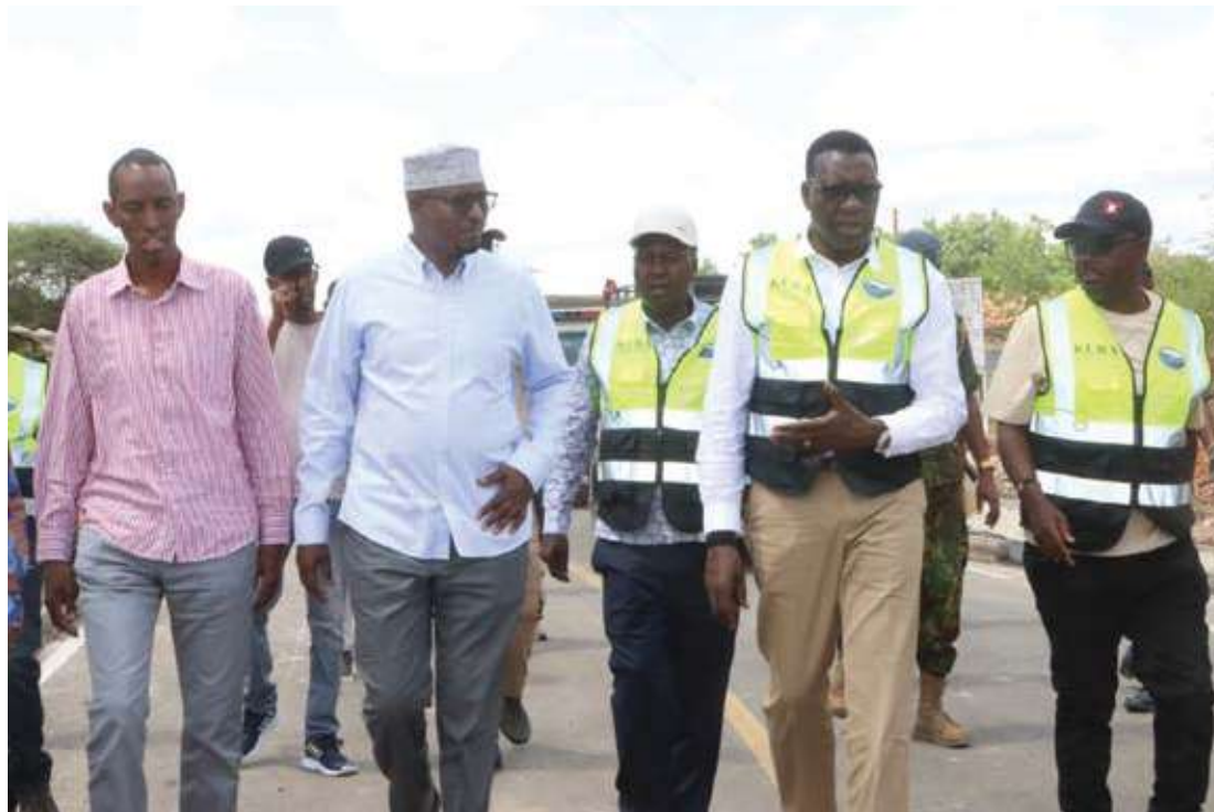
Roads and Transport Cabinet Secretary, Davis Chirchir (second from right), Wajir Governor Ahmed Abdullah and Deputy Governor, Ahmed Muhumed, inspecting ongoing road projects in Wajir town alongside officials from the Kenya Urban Roads Authority ahead of the Madaraka Day celebrations scheduled for June 1.
