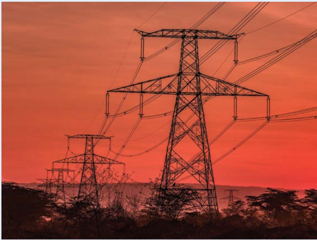
KETRACO transmission lines.
