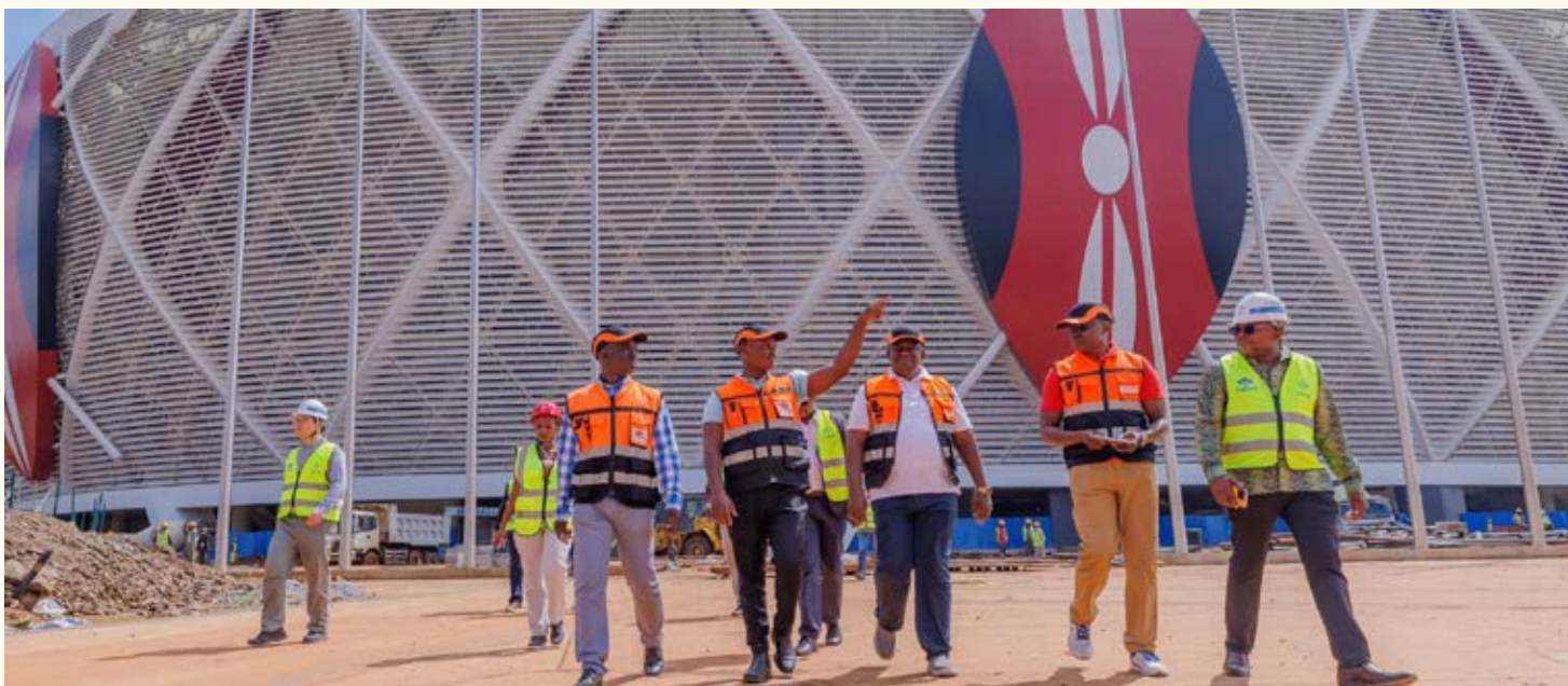
Sports Cabinet Secretary Salim Mvurya (third right) at the Railla Odinga International Stadium located at the Talanta Sports Complex during an inspection tour. The stadium is 91 per cent complete. Mr Mvurya said its three training pitches are 87 per cent complete, while key final works including landscaping, lighting, fencing and power connectivity continue to progress steadily.
