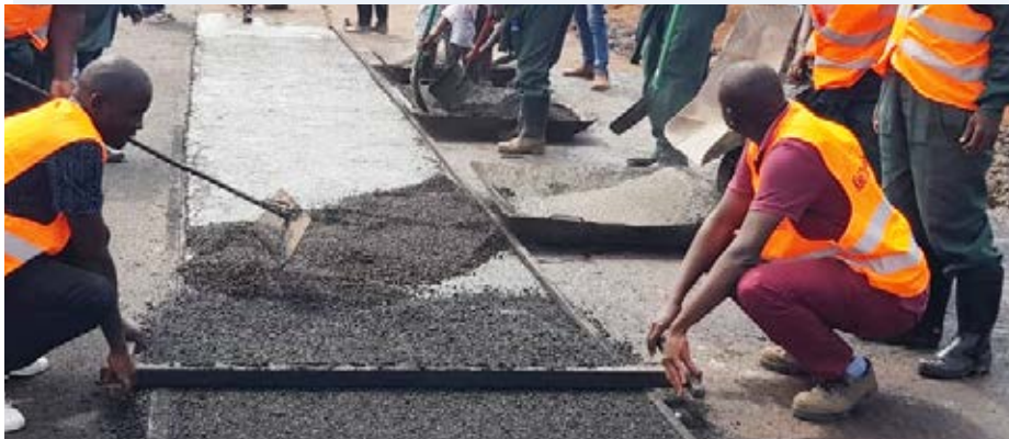
KIHBT Practical training on Construction of Low Volume Sealed Roads.
