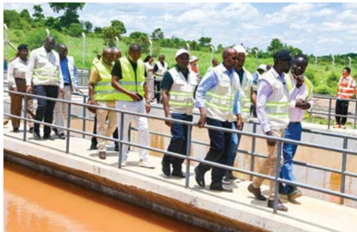
Water, Sanitation and Irrigation Cabinet Secretary Eng Eric Muriithi Mugaa, leading the team, (in a black cap) accompanied by Tanathi CEO Sammy Naporos and Mwala MP Vincent Musyoka during the inspection of ongoing Mwala Cluster Water Project in Machakos County.
