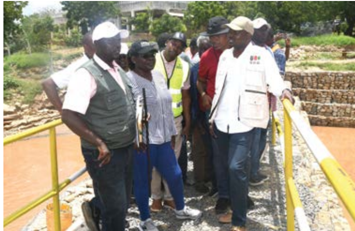
Head of Government Delivery Unit Sitali Olando (right) and Coast Regional Commissioner Rhoda Onyancha (centre) lead multi-agency team on an inspection and verification tour of critical infrastructure within the Galana Kulalu Food Security Project. PHOTO BY BENEDICT WASICHE
