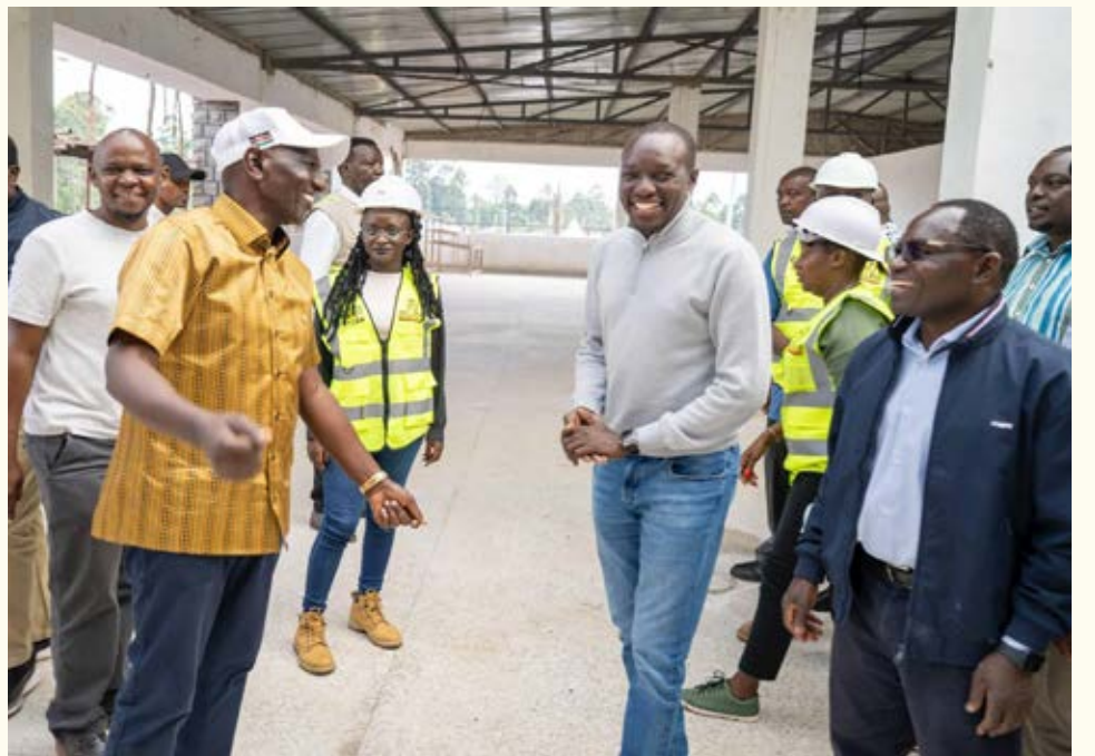
President William Ruto (left), Governor Simba Arati (centre) and Broadcasting and Telecommunications PS Stephen Isaboke (right) in Bomachoge Chache, Kisii County. The President launched the construction of 11km Sameta-Egetuki-Ikoba Road and inspected the ongoing construction of Egetuki Modern Market, among other projects.
