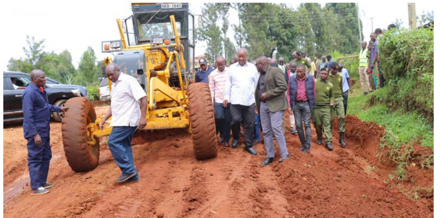
Nyamira Governor Amos Nyaribo inspects a county road under construction as he improves the road network in the region. PHOTO/KNA
