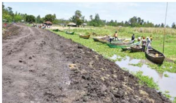
Ongoing West Kano Kanyagwal Flood Control Project that involves construction of a 1.5-metre-high dyke spanning 3.5 kilometres and a footbridge in Ogenya Sub-location, Kisumu County.
