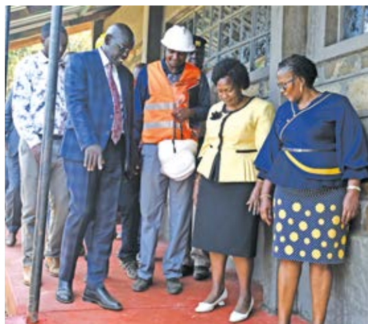
Principal Secretary, State Department for Basic Education, Dr. Belio Kipsang (left) at Sulgwita primary in Turi, Molo sub-county to inspect the construction progress of grade nine classes.
