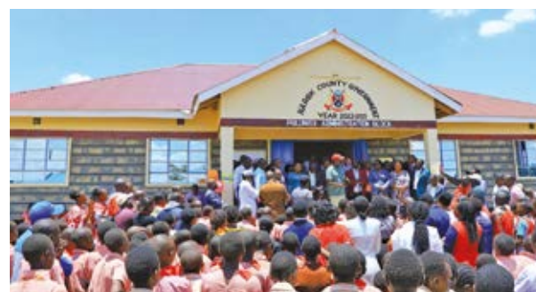
A new administration block commissioned at Pulunga Primary school within Narok township ward
