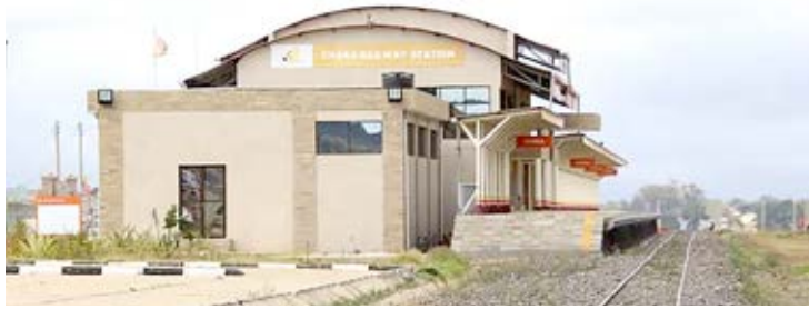
Chaka Train Station in Nyeri county. The Ministry of Roads and Transport is seeking views from members of the public on the Railways Bill 2024 which is seeking to open-up the railway infrastructure to private operators.
