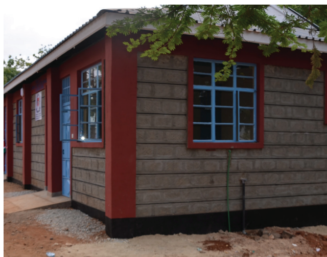
A glimpse at the modern dining hall funded by NFDK at Mwanyambo Special School for the deaf.
