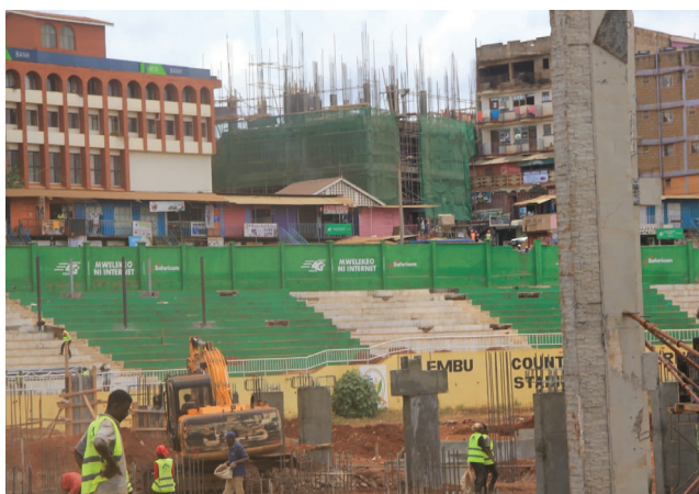
The ongoing construction works at Embu stadium
