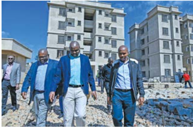
Eastern Regional Commissioner Paul Rotich leads the National Government Coordination Secretariat on an inspection of NHC Affordable housing in Embu.
