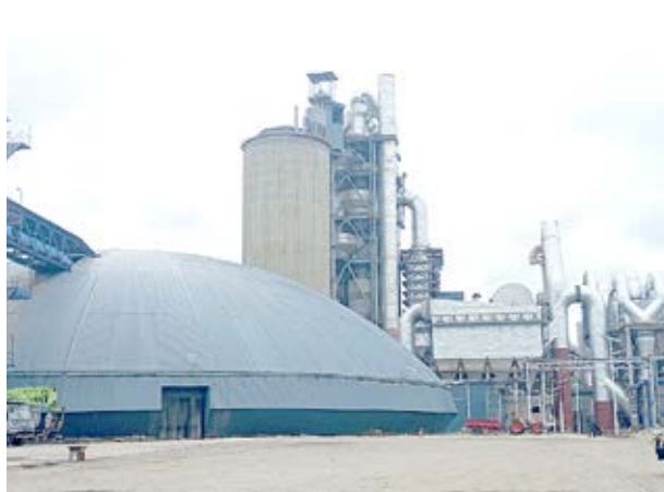
A side view of the Clinker Production Company at Sebit constructed by Devki Group of Companies in Kipkomo Sub County in West Pokot County. PHOTO: ANTHONY MELLY
