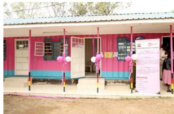
A section view of the Kasagam Police Station Child Protection Unit launched by Gender, Culture, Arts and Heritage CS, Aisha Jumwa. The two facilities were built through funding from the Kisumu County Office of Woman Representative NGAAF kitty.
