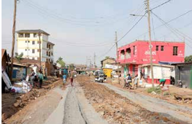
Ongoing upgrading of Kisumu’s Manyatta slums by KISIP2
